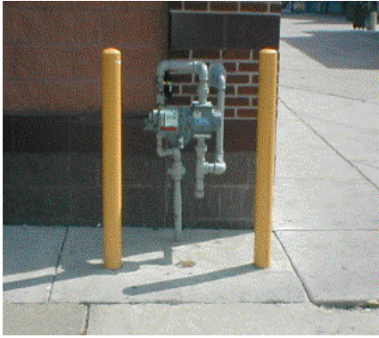
Bollards Installed to Protect
